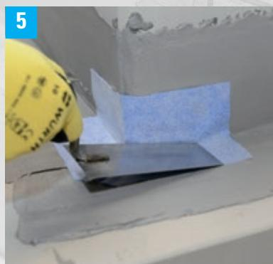
5 Embed MC-FastTape AE (outer corner) or MC-FastTape IE (inner corner) in the first fresh layer.
