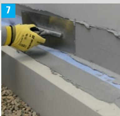
7 Embed MC-FastTape and apply the last waterproofing layer.
