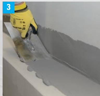
3 Apply scratch coat and allow to dry.
