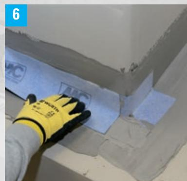
6 Apply MC-FastTape so that it overlaps at the inner or outer corner by at least 10 cm. Use the waterproofing compound as an adhesive for the connection.
