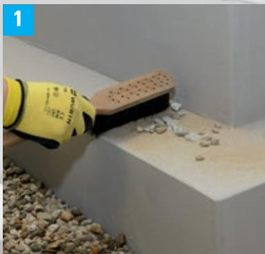
1 Clean the substrate. Fill pores and cavities > 5 mm with a suitable mortar.
