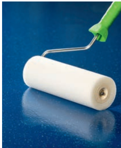
Sealing after strewing with chips
