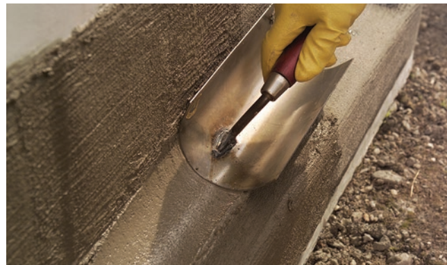
Mineral fillet created with a rounded trowel
