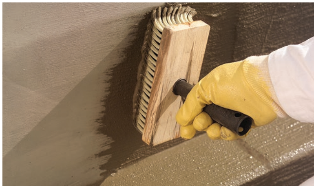
Applying waterproofing slurries in the shoulder area
