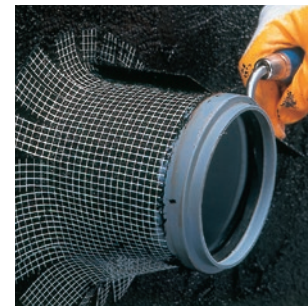
Trowelling-on the second layer of Nafuflex
