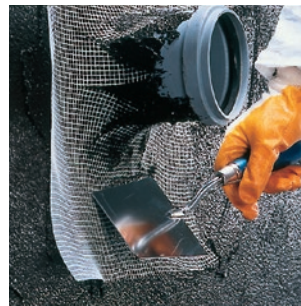
Incorporation within the first layer of Nafuflex
