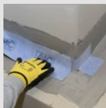
Apply MC-FastTape so that it overlaps at the inner or outer corner by approx. 10 cm.
