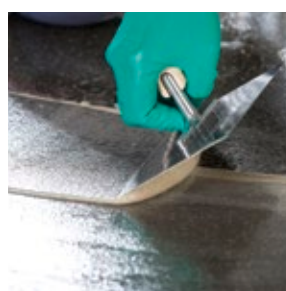
Scratch and levelling coat MC-Floor TopSpeed SC with sand filler
