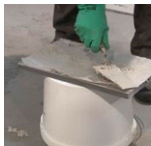
Adhesive coating over the full area
