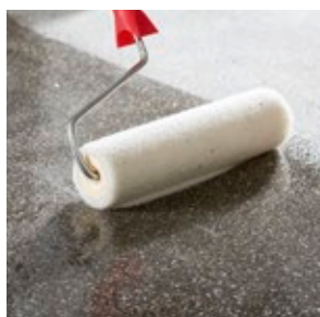
Primer and bond coat MC-Floor TopSpeed SC
