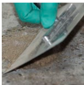
Filling cracks and crevices MC-Floor TopSpeed SC with sand filler
