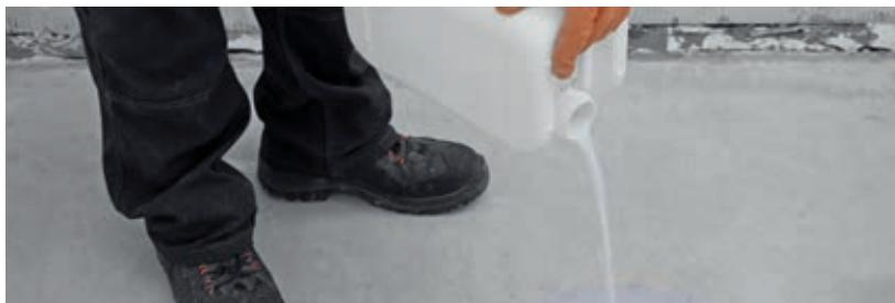
MC-Estrifan SI is evenly applied with a Gloria spraying pump or MC-Spezialspritze in a crosswise and lengthwise pattern on the matt damp surface. The treated area must be kept moist until the reaction has been completed (approx. 60 minutes). If MC-Estrifan SI is used as wet curing, the surface has to be kept wet for the minimum of 24 hours.
